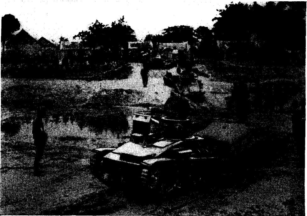
Figure 20.—Model 92 (1932) tankette with tracked trailer.
